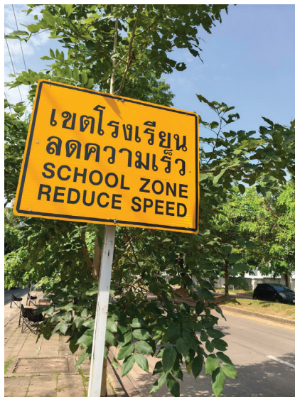
Figure 9 Example of Supplementary Advance Warning Sign Installation Prior to Pedestrian Crossings near School Zones
